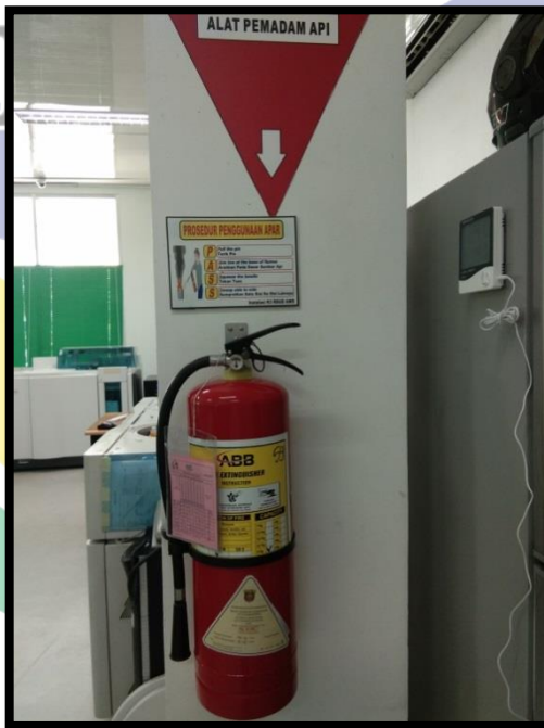
Gambar 6. APAR Jenis Powder di Laboratorium Kimia Klinik RSUD Abdul Wahab Sjahanie Samarinda
